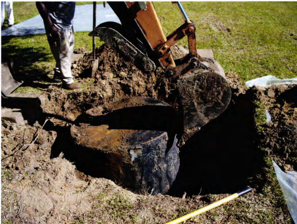
Picture 2: UST 469Dogwood removal in progress .
